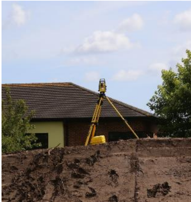
Robotic Total Station
