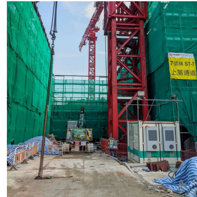
Enertainer powering a tower crane lifting a heavy MiC module
