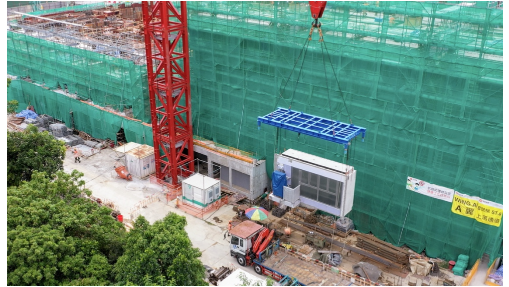
Enertainer powering a tower crane lifting a heavy MiC module
