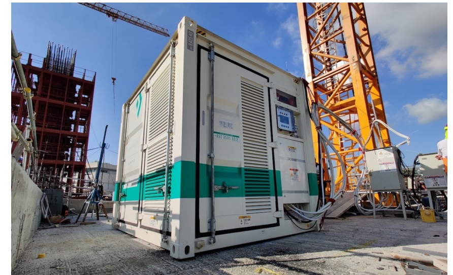
New method: Enertainer, clean battery energy storage system
